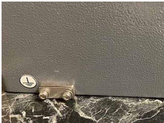
External Grounding Connection Point
